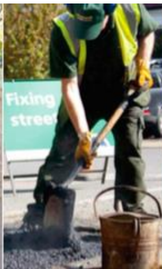
Repairing roads and pavements
