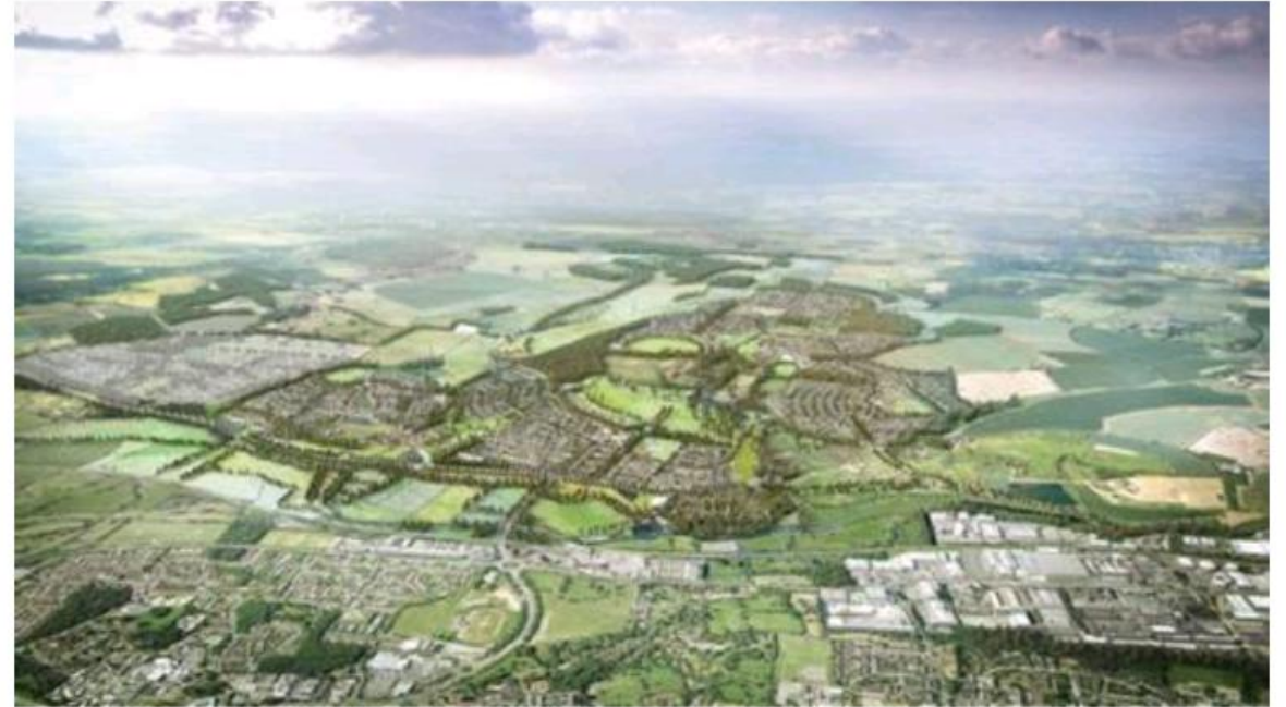
Aylesbury Vale GT – Highway Infrastructure £9.5m
