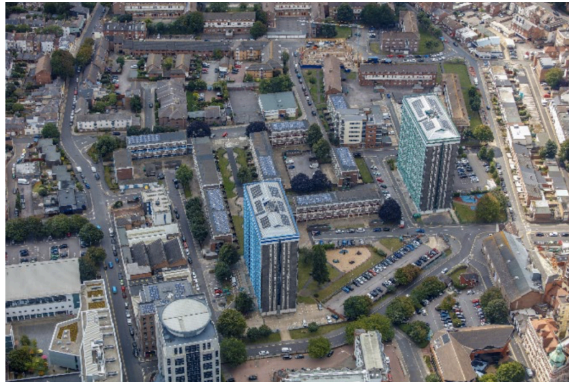
Aerial view of Horatia House and Leamington House
